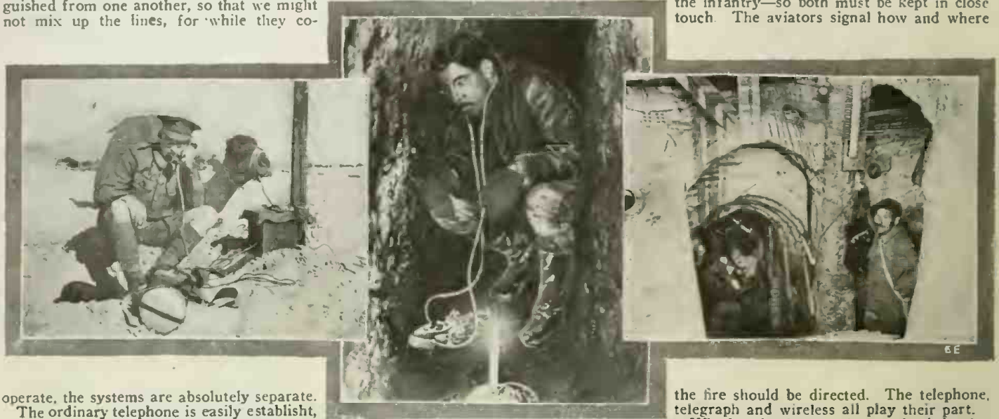
Photos from Central News Photo Service
